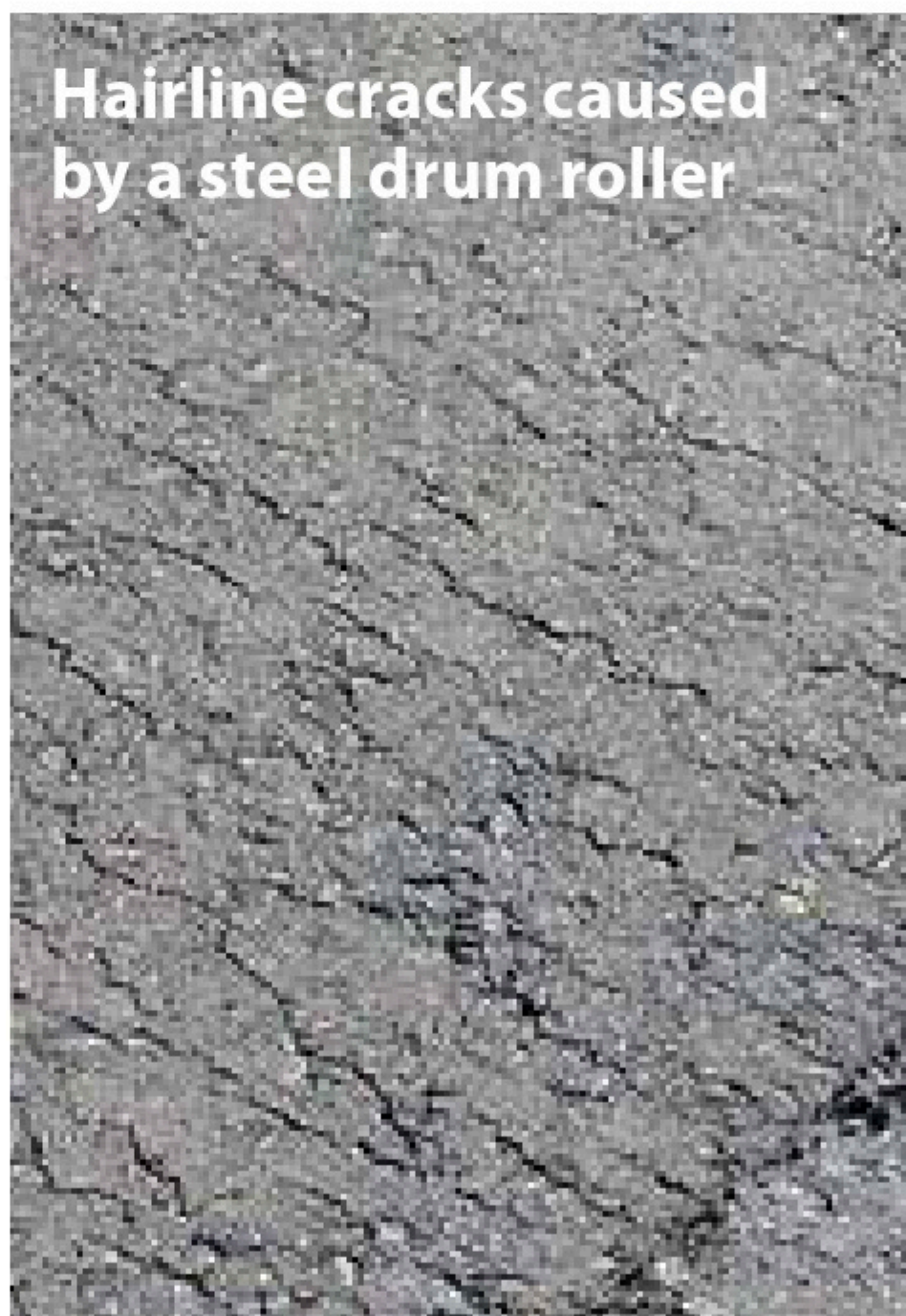
Fig 4. Remove hairline cracks from HMA pavement
