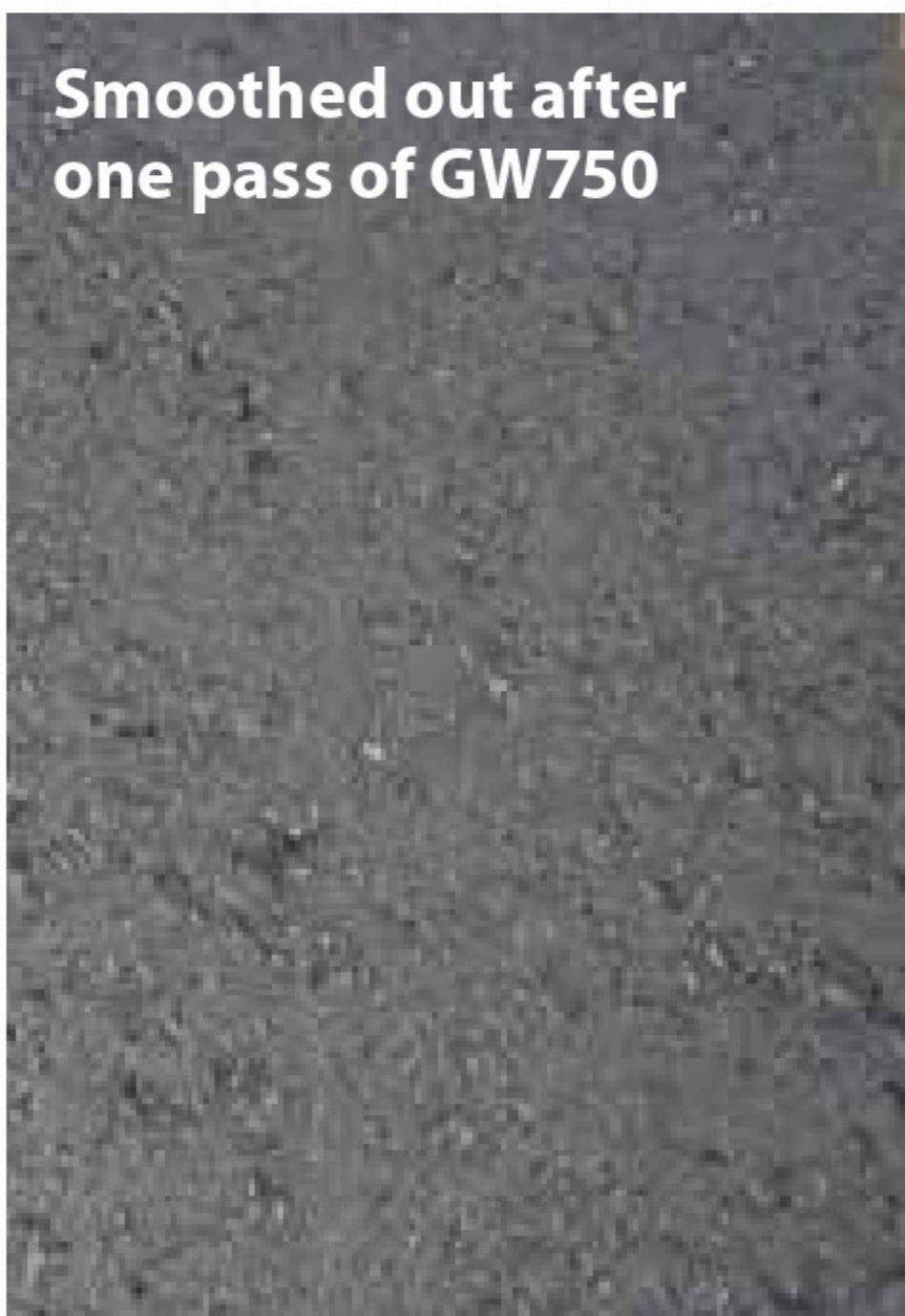
Fig 4. Remove hairline cracks from HMA pavement
